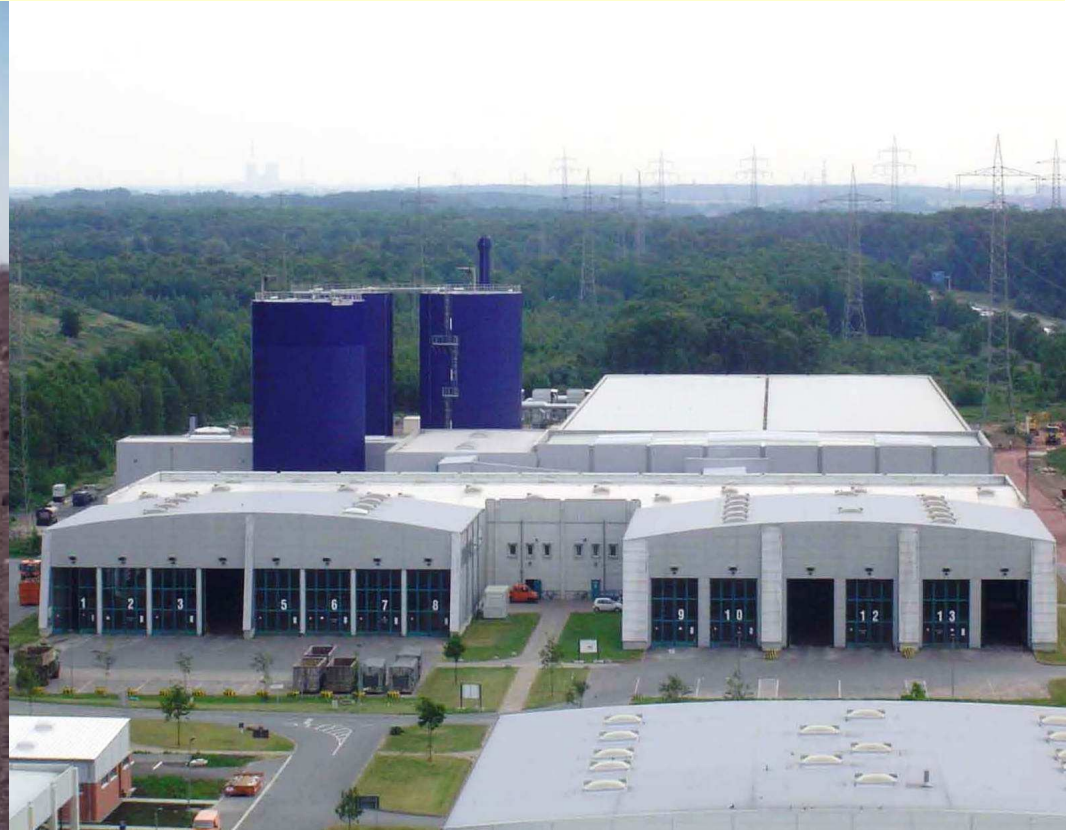
Fully encapsulated, anaerobic MBT with RDF production, source: aha Hanover (regional public enterprise for waste disposal services)
